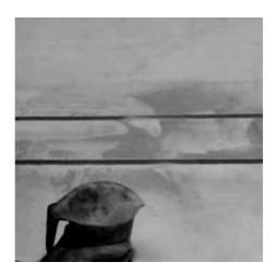
2. Distribute the sand evenly. Observe the minimum dimension w for the remaining depth of the groove.
