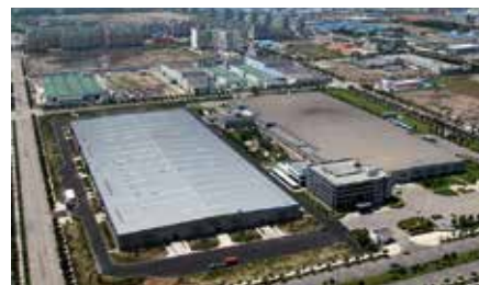
SEW-EURODRIVE Co., Ltd., Tianjin, China
